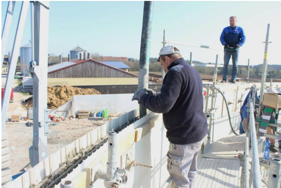
Figure 19. concreting the tank wall
