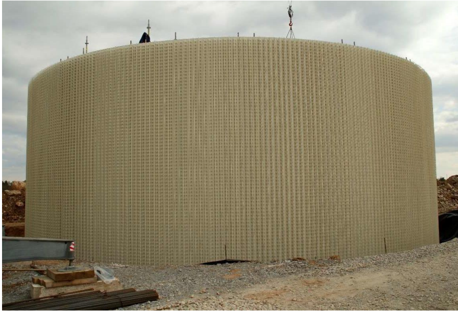
Figure 11. closed inner formwork
