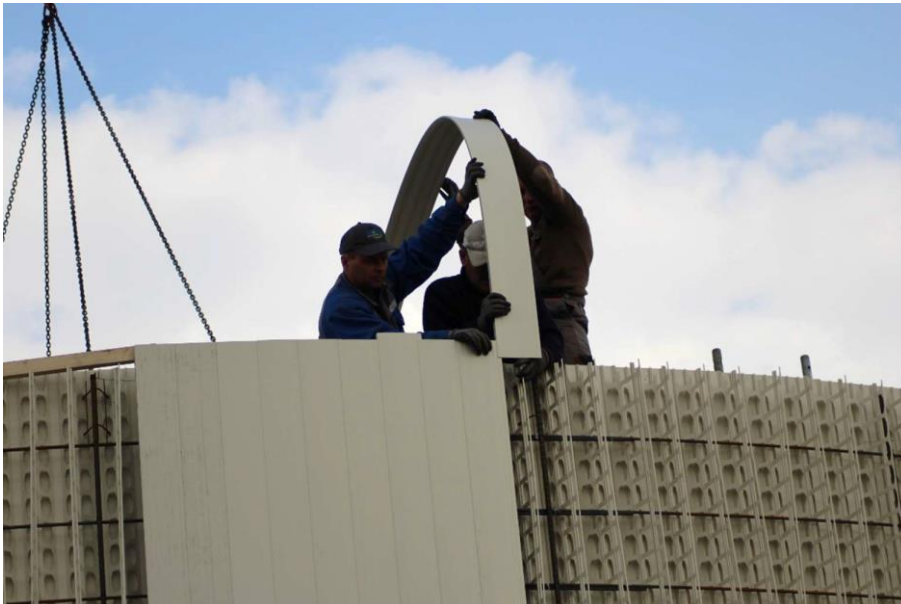
Figure 16. assembly the outer panels
