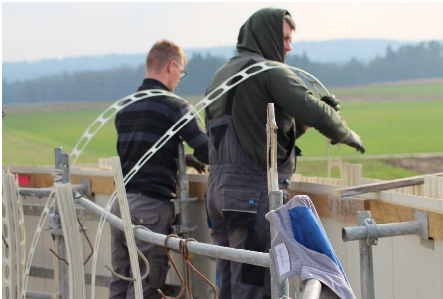
Figure 17. mounting 45° stiffeners on outer panels
