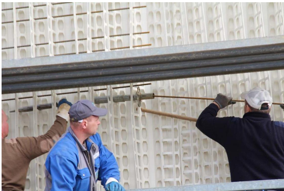
Figure 12. insertion of the horizontal reinforcing bars
