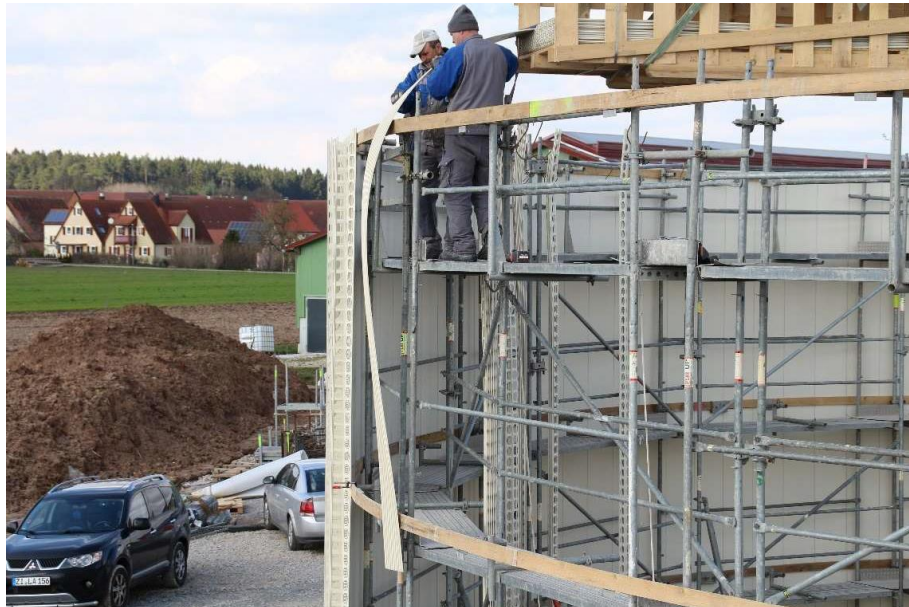
Figure 5. mounting inner panels
