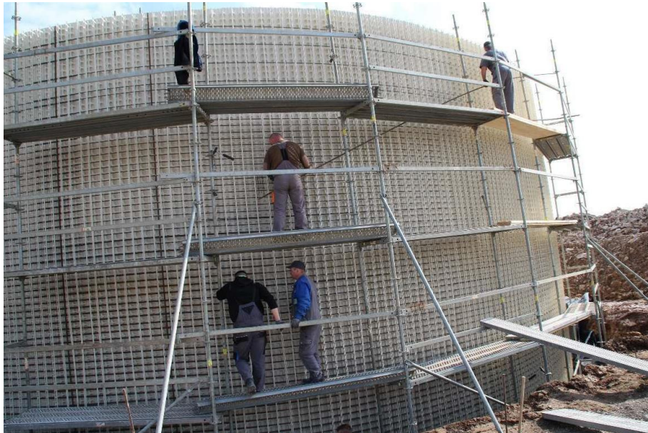
Figure 13. assembly of the vertical reinforcing bars.
