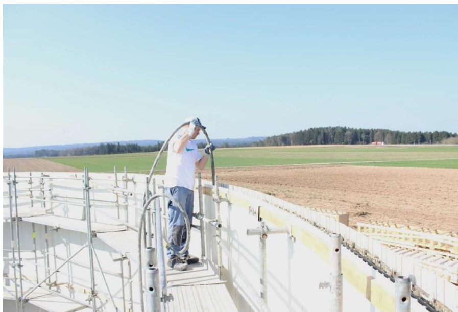
Figure 20. compacting the concrete with vibratory flasks.
