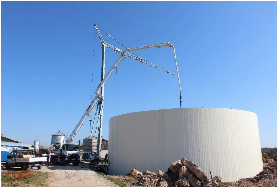
Figure 21. filling the formwork with concrete
