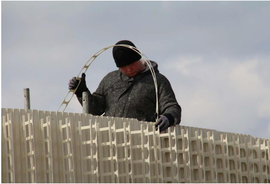
Figure 9. 45° stiffeners assembly
