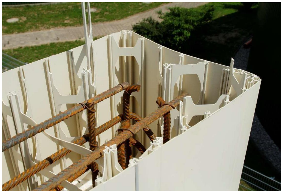
Figure 24. execution of the wall ends
