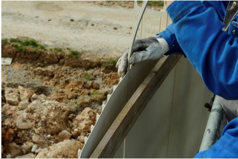
Figure 7. mounting connector for inner panels
