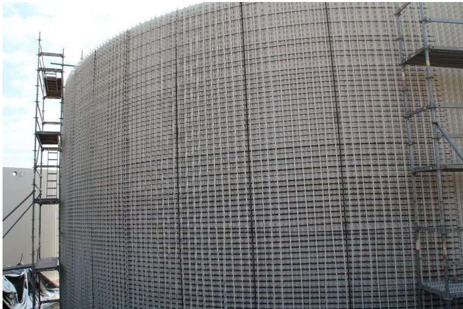
Figure 14. finished reinforced tank wall
