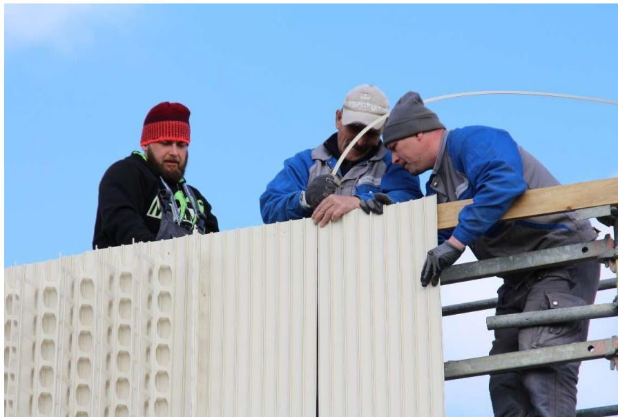
Figure 6. mounting connector for inner panels
