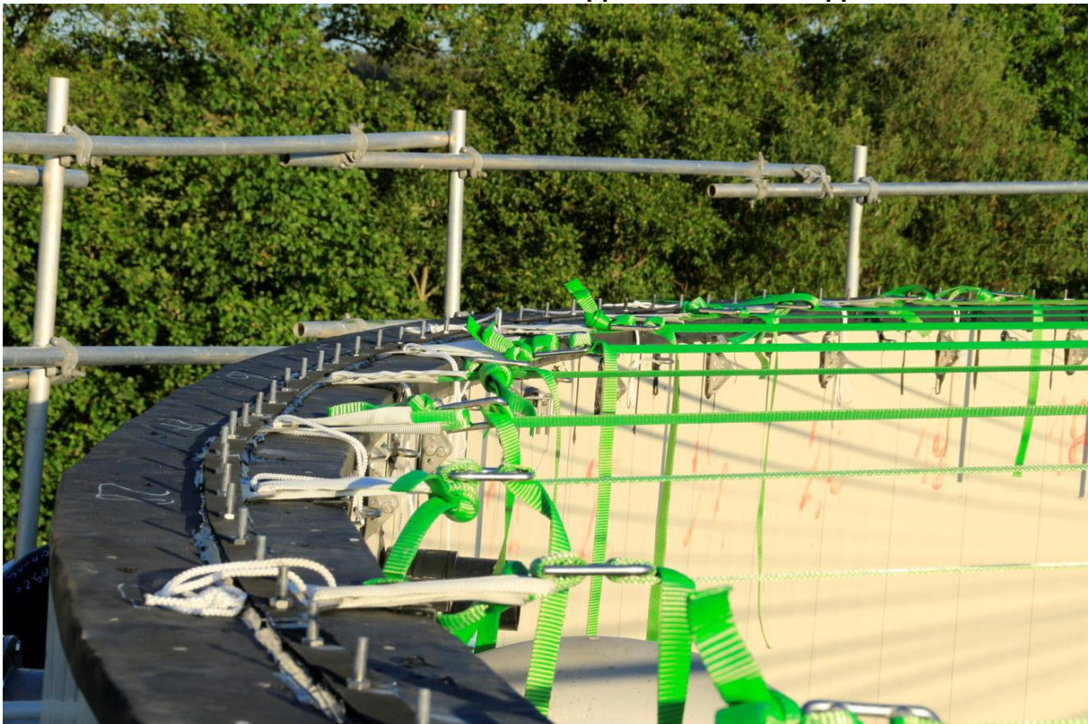
Belts are tensioned over the center support towards the opposite rail
